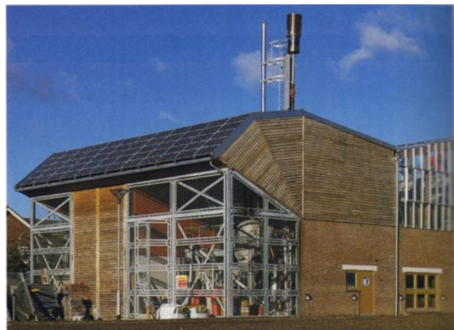
Combined Heat and Power Plant Source: http://www.bedzed.org.uk
