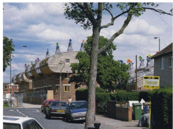
The decision to face the buildings south means that the main public facade is a series of building edges, rising and falling like waves and adding interest to the street. Source: Gregory, p. 44
