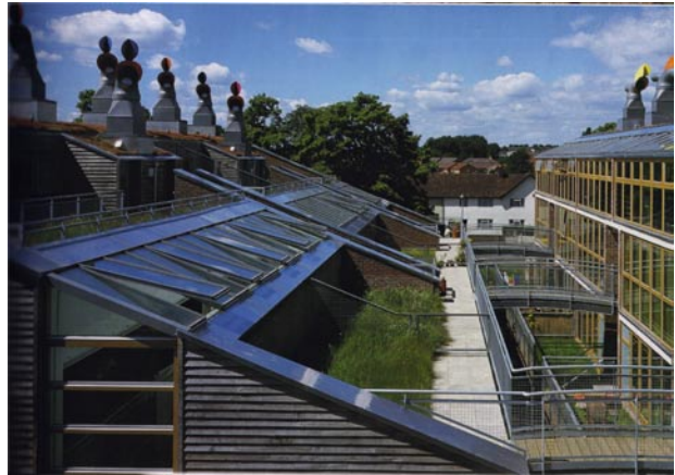
BedZED gardens are located on the sloping north side of the buildings. Some are reached by sky bridges from units on the other side of the mews. Source: Gregory, p. 47
