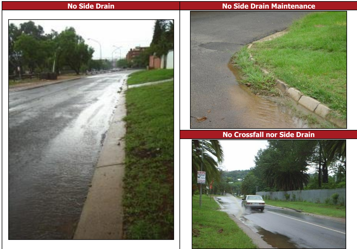
Figure 33. Poor Surface Drainage (from SANRAL Drainage Manual)
