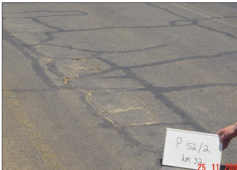
Figure 27. Pumping of Stabilized Base
