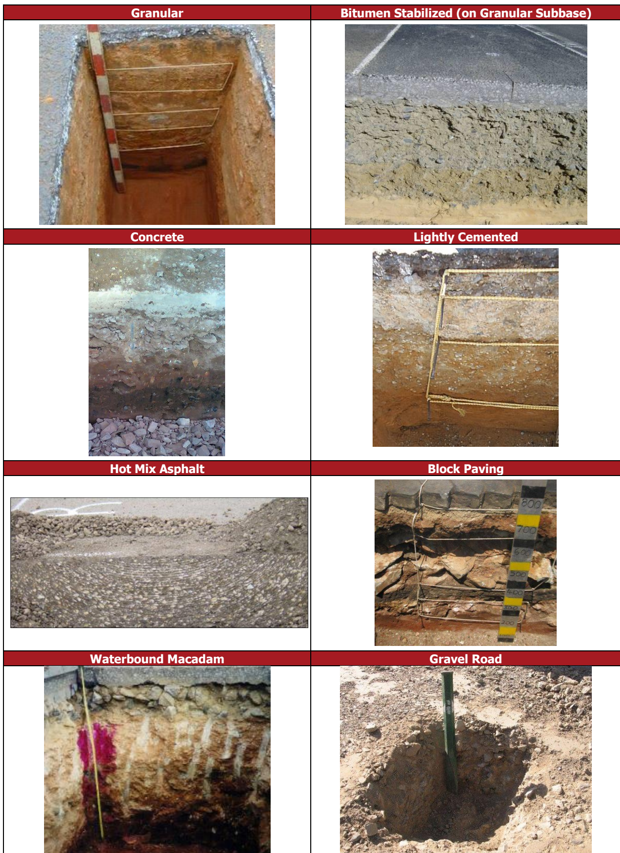
Figure 4. Example Cross-sections of the Typical Pavement Materials
