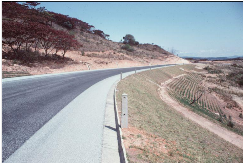
Figure 11. Drainage Bench
