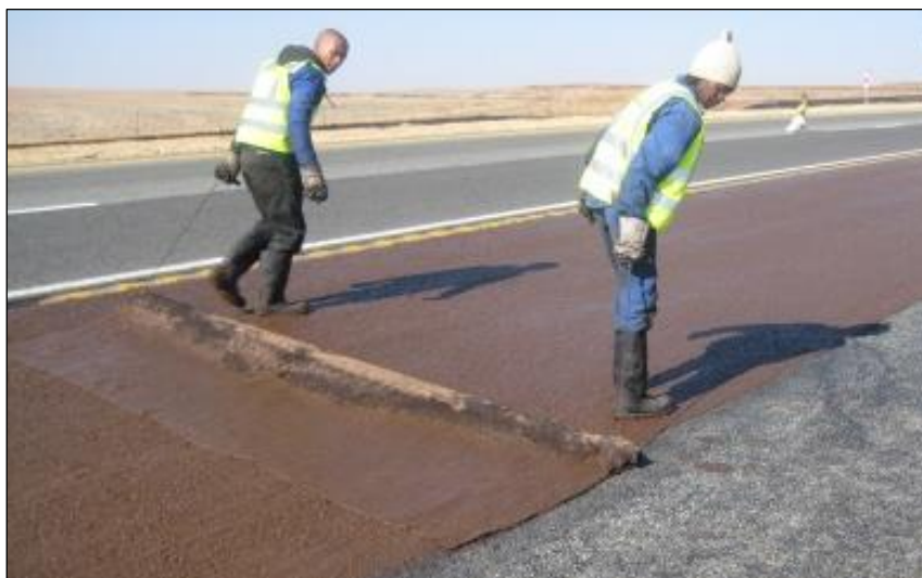
Figure 41. Application of a Slurry
