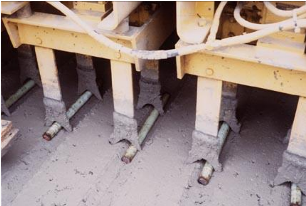
Figure 51. Inserting Dowel Bars
