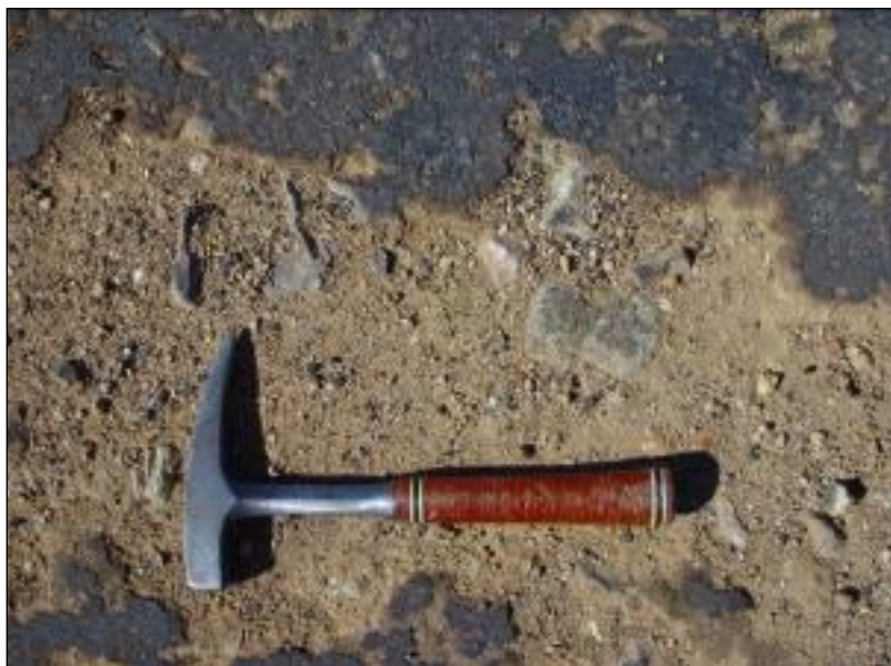
Figure 16. Loss of Adhesion Between Base and Seal
