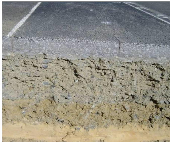
Figure 28. BSM-Foam Base Layer on Crushed Stone Subbase
