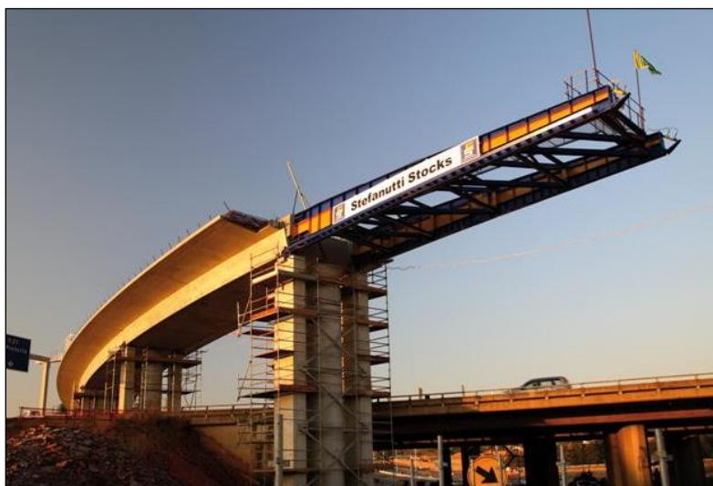
Figure 42. In Situ Incremental Bridge Construction
