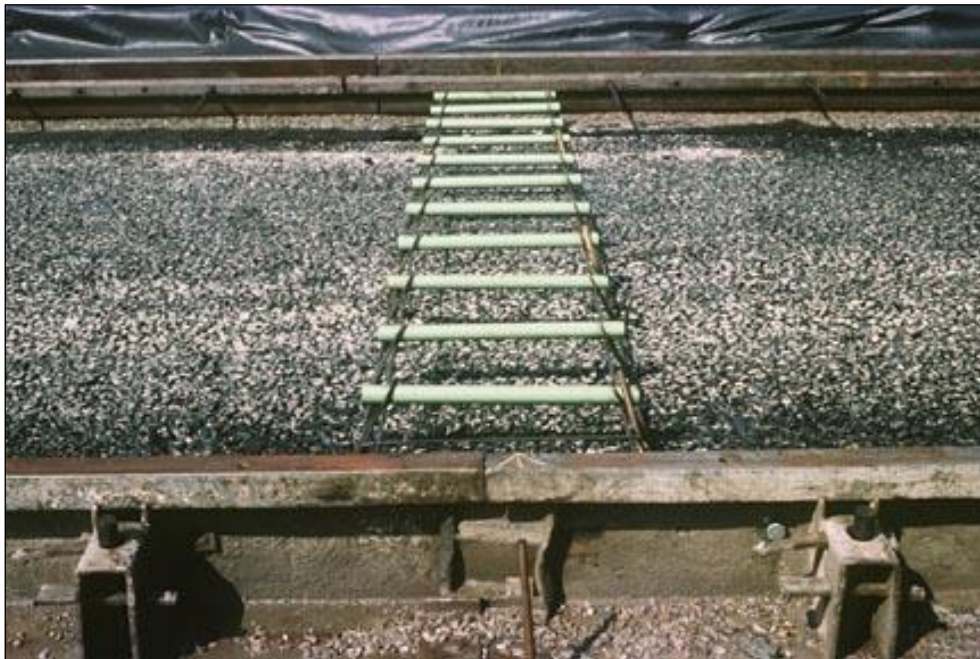
Figure 45. Installation of Dowel Bars
