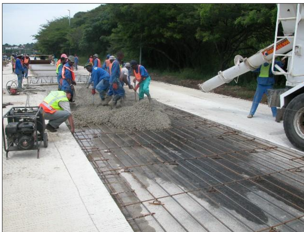
Figure 47. Constructing a Continuously Reinforced Concrete Pavement
