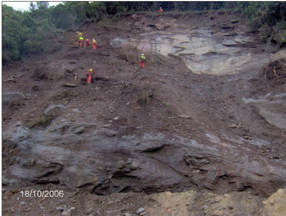
Figure 21. Slide on Unfavourable Bedding Plane
