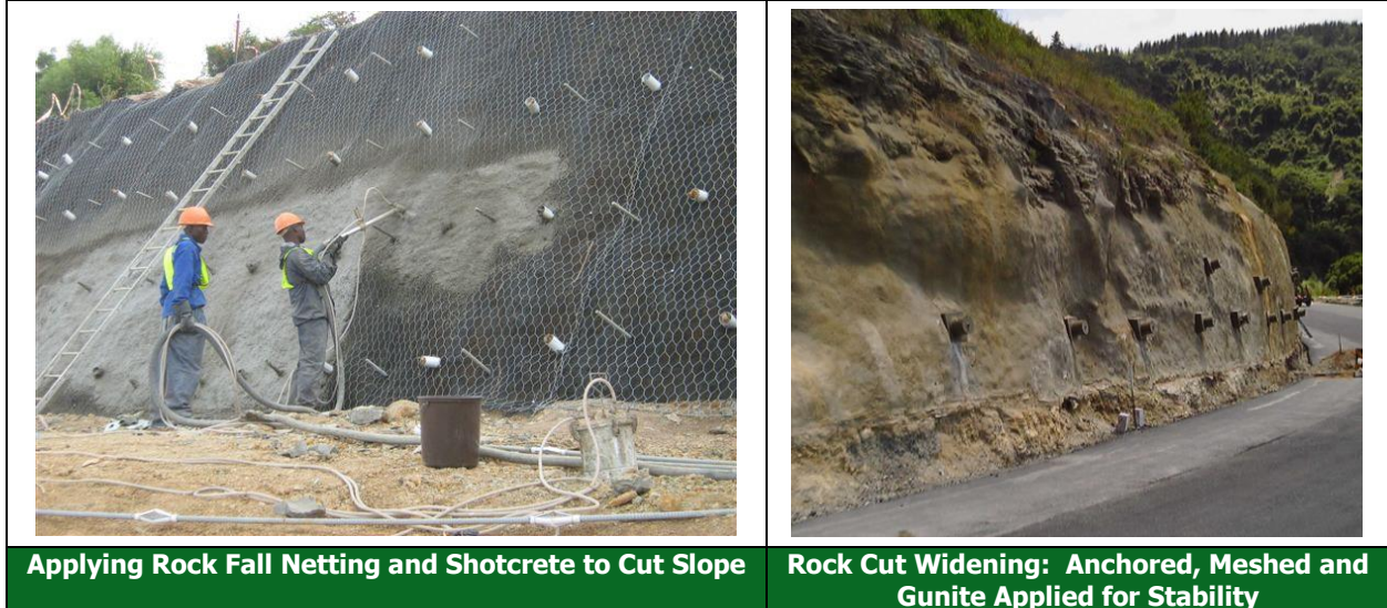
Figure 18. Applying Rock Fall Netting and Shotcrete to Cut Slope
