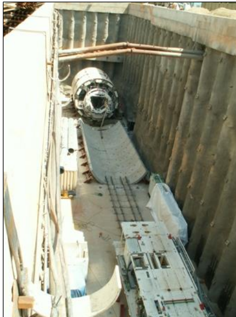
Figure 40. Tunnel Boring Machine at Entrance to Tunnel at Gautrain's Rosebank Station
