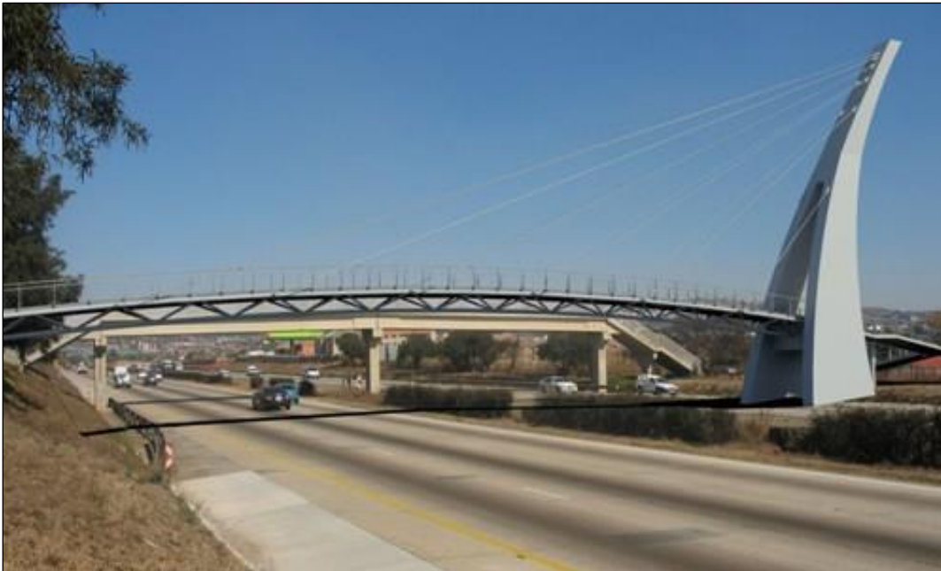
Figure 35. Pedestrian Bridge Over the N1
