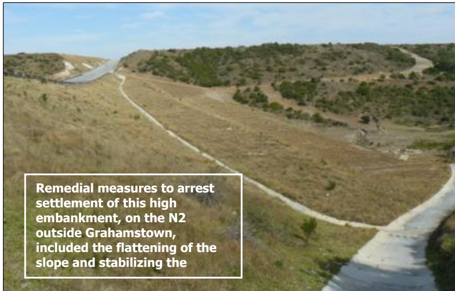
Figure 8. Preventing Settlement on High Embankment
