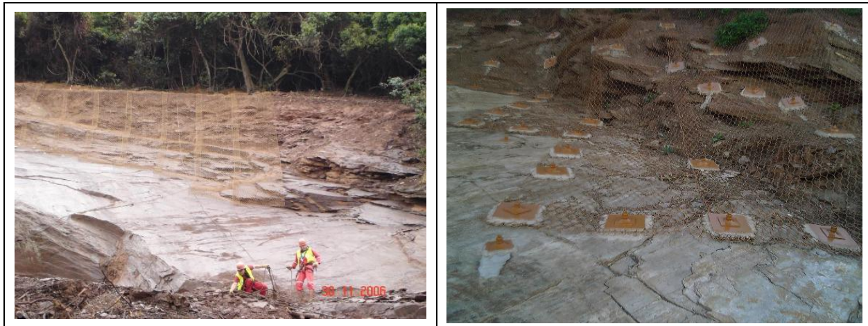
Figure 22. Doweling as a Stabilization Method
