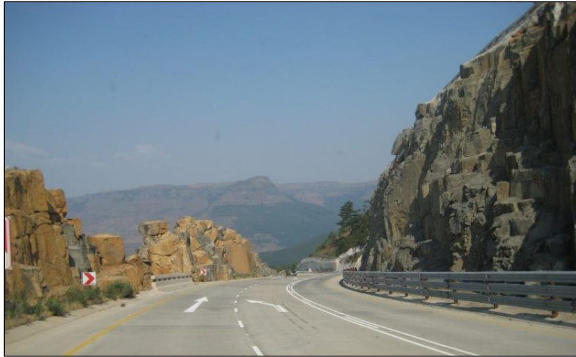
Figure 14. Example of a Road Cut in Rock
