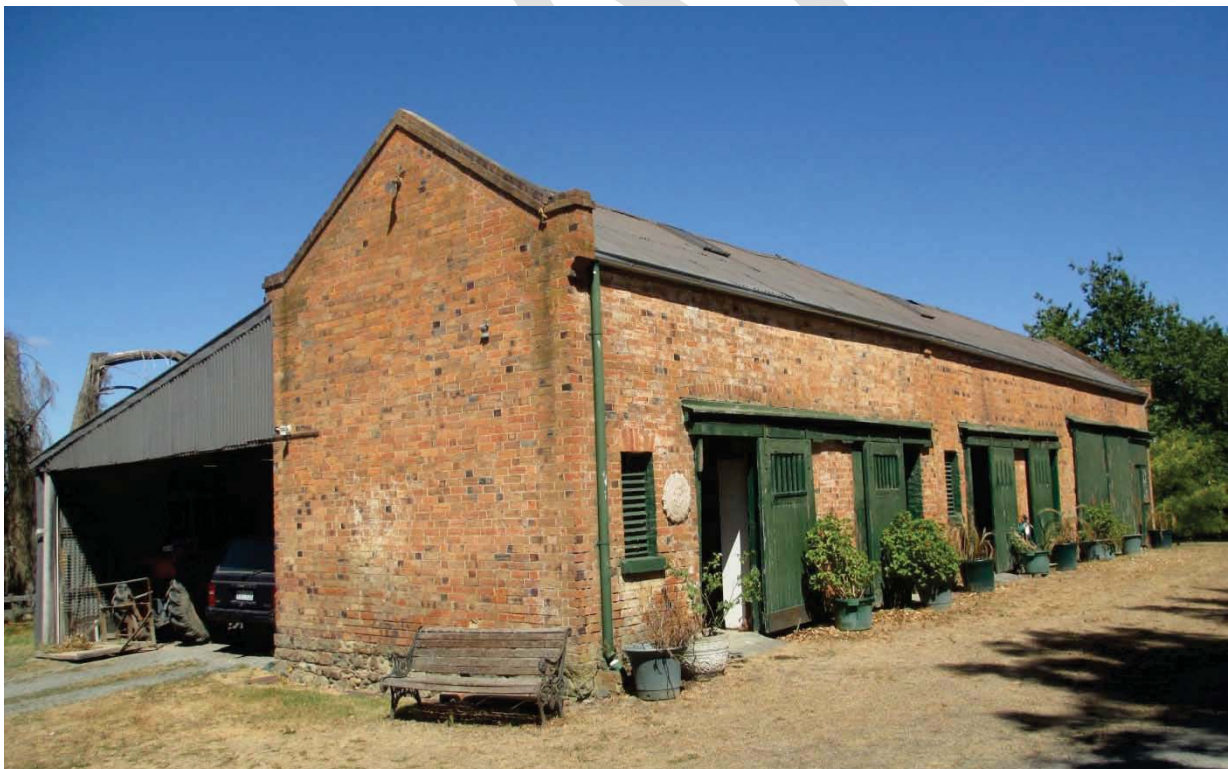
Historic stables building, with lean-to at left.
