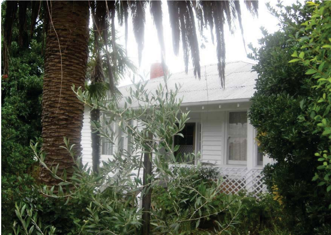
Detail of the front verandah and entry.
