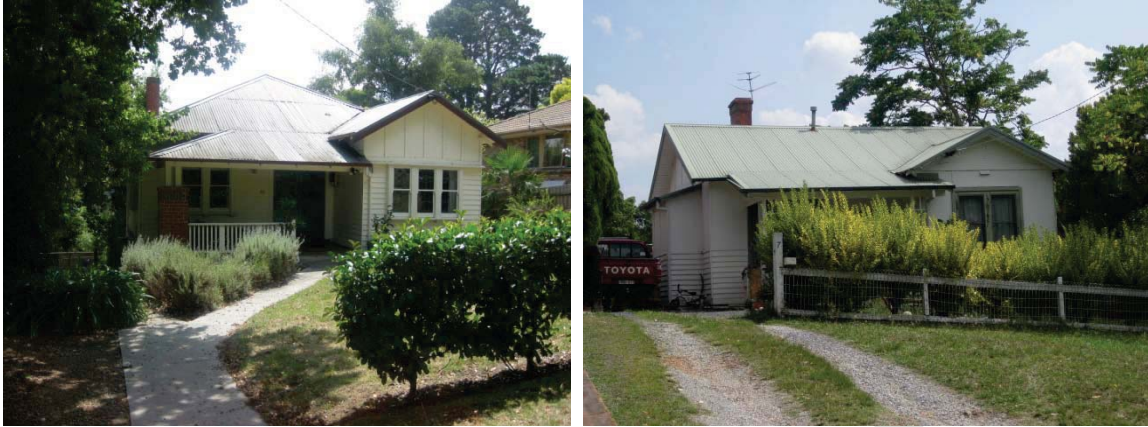
Figure 23 Variants on the Californian bungalow form – 41 Symons Street, c. 1930, constructed of timber and with a hipped roof; and 7 Manse Street, c. 1940, constructed of timber and cement sheet and with a transverse gable roof. Both are graded as 'contributory'.
