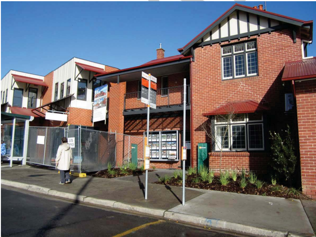
Figure 24 Former residence and shop building, to the south-west corner of Green and Nicholson streets, viewed from Green Street ('contributory'). The additions to the left are of recent construction.
