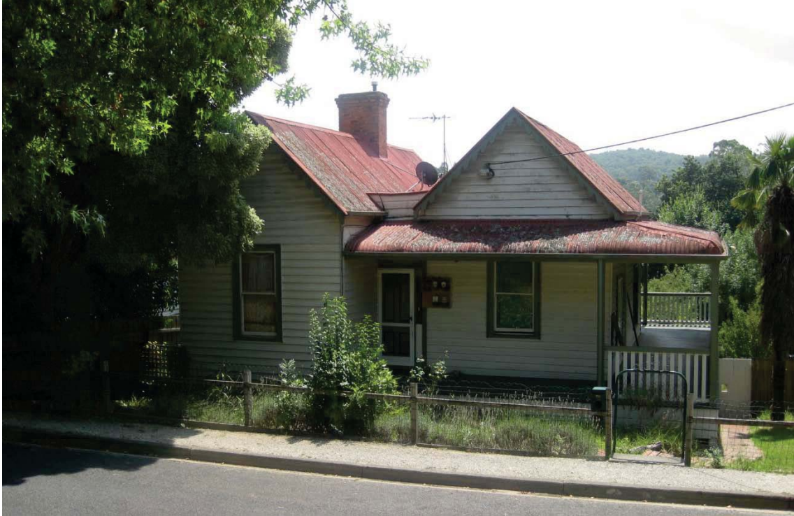
Figure 17 17 Symons Street, c. 1900, an unusual double-gabled cottage with a return verandah and large lower level, on a sloping block to the north side of Symons Street. The property is graded as 'contributory'.
