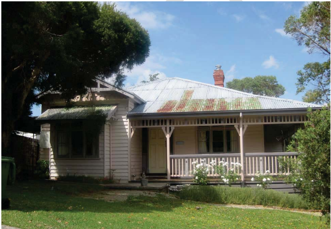
View of subject property from Westmount Road.
