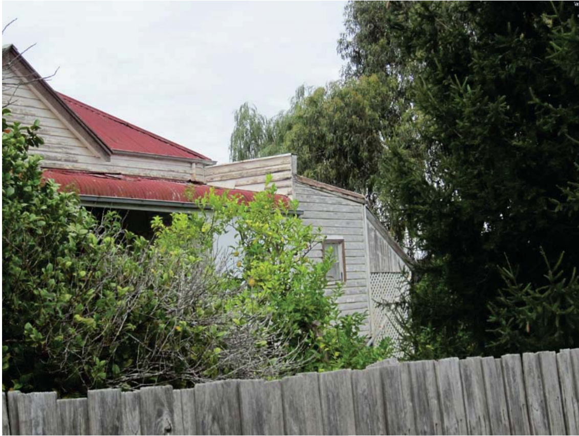
North elevation and verandah enclosure to the rear.
