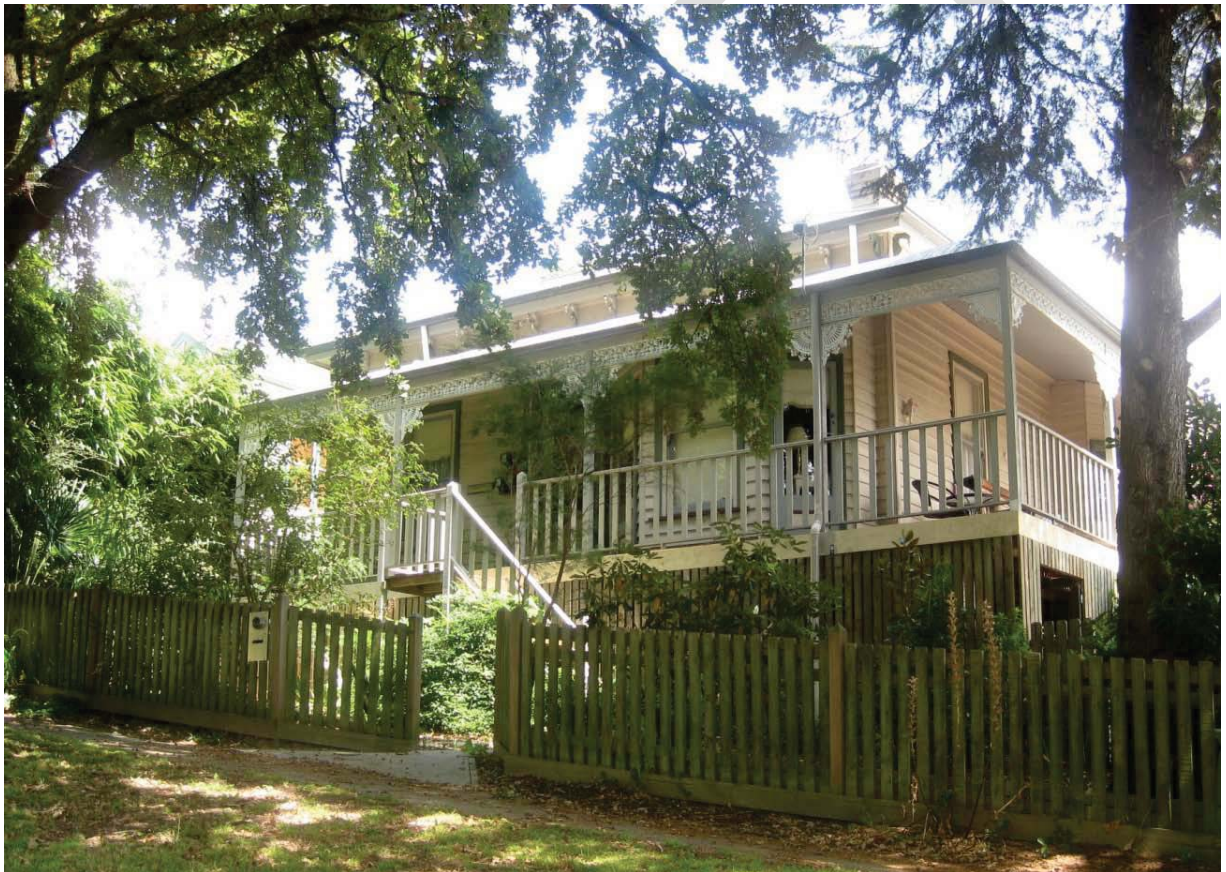
Figure 20 1 Church Street c.1900, a late Victorian villa with canted bay windows, graded as 'contributory'.
