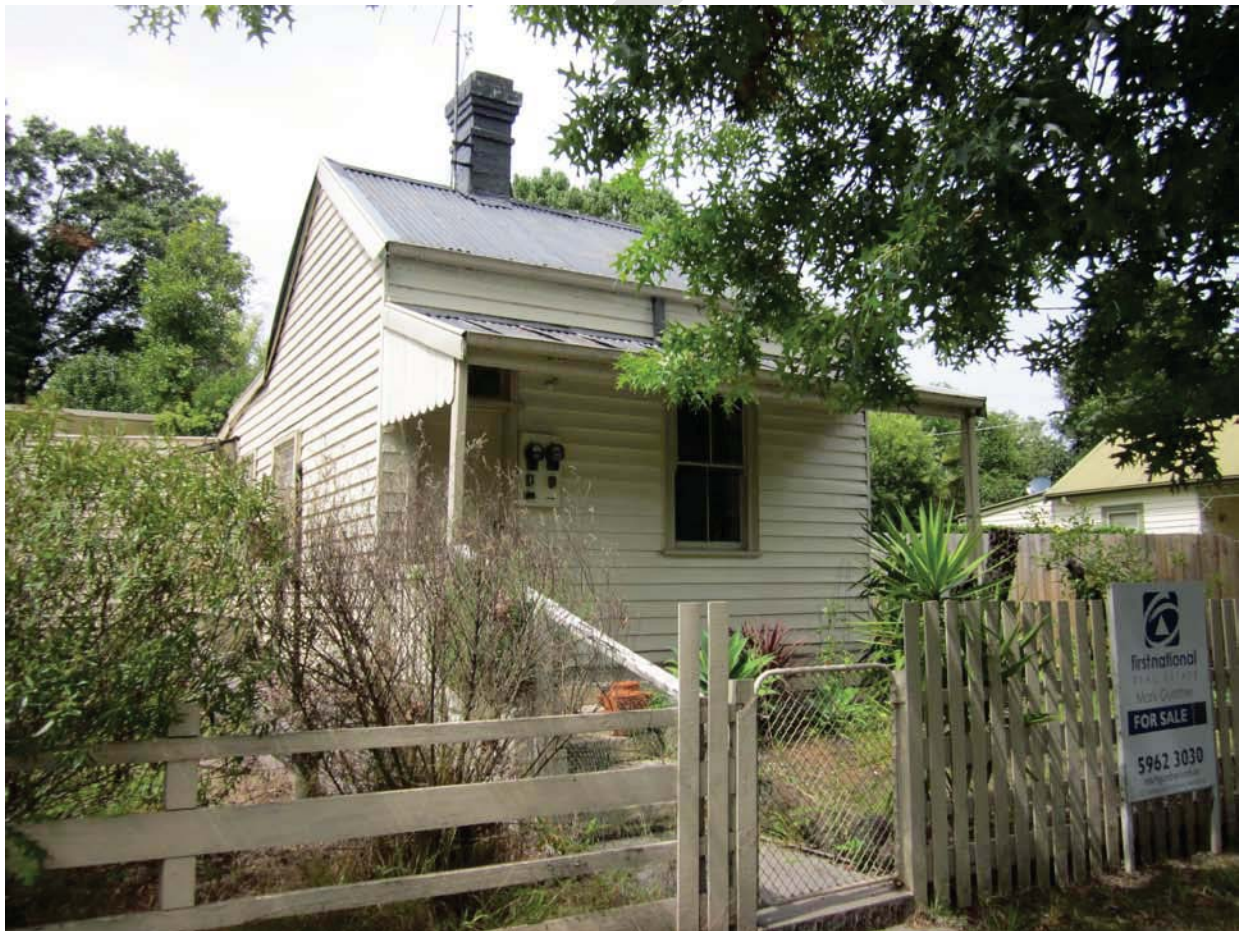
Façade and part of the east elevation of the cottage.
