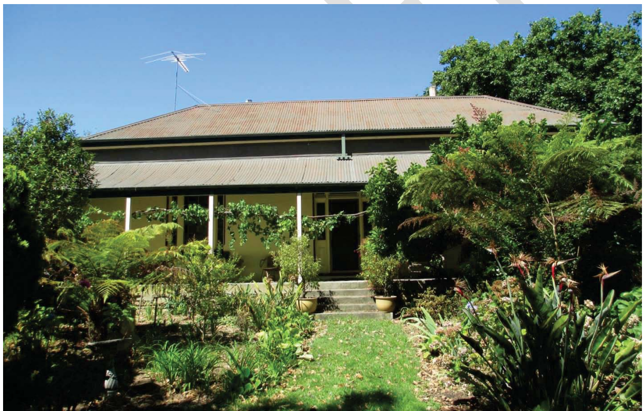
North elevation of residence.
