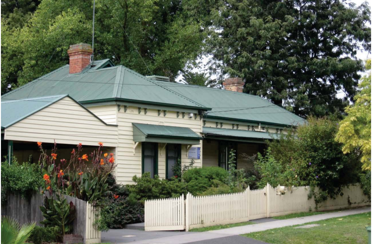
Figure 14 Former Inglenook Guest House, 2 Green Street, c.1891 graded as 'contributory'. The two phases of its construction are evident in the two main building bays.
