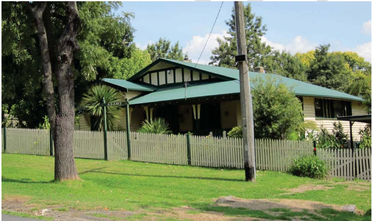
Subject property as seen from Harker Street.
