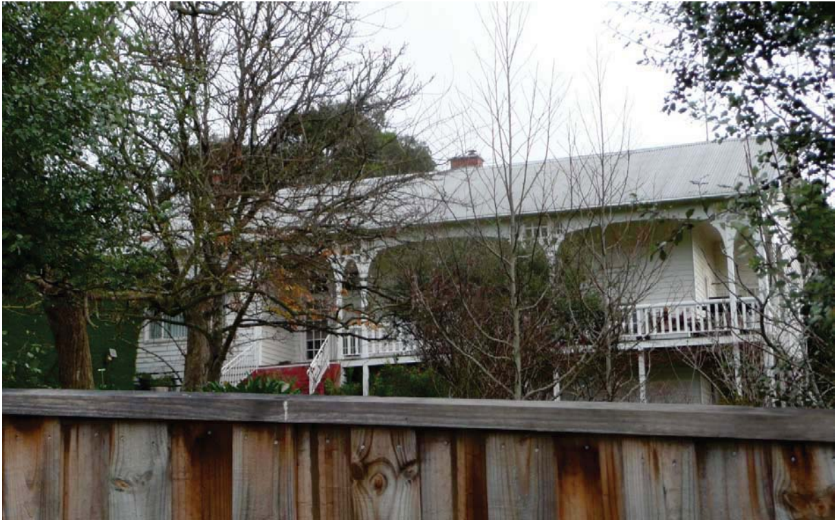
Figure 25 Neangar , 27-29 Crowley Road, 1924-25. This property is graded as 'significant'.
