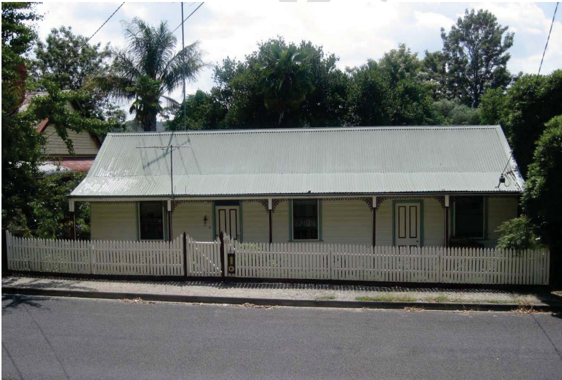
Figure 18 31 Symons Street, a Victorian-era villa, with a pattern of door and window openings which suggests it may have originally been a pair of houses. Graded as 'contributory'.
