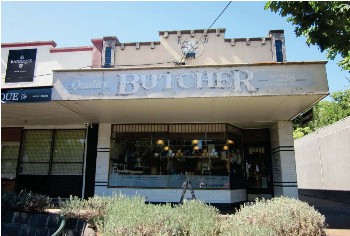
Figure 21 Butcher shop, 258 Nicholson Street, assessed as 'contributory' to the precinct.
