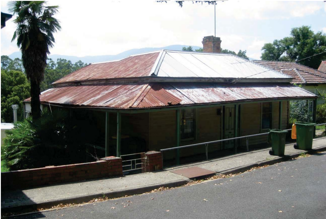
Figure 16 13 Symons Street, c. 1900, a double-fronted Victorian cottage, set close to the street on the north side of Symons Street, graded as 'contributory'.
